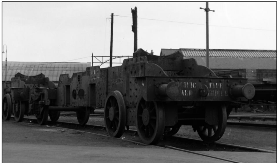
This rather unusual picture depicts two long scrapped locomotive chassis. Having been stripped down they have been put to good use to transport boilers around the works.
